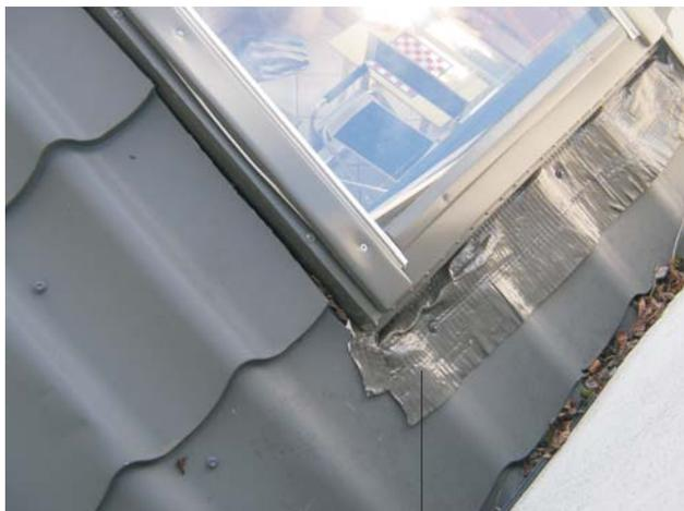
Badly fitted/ damaged Velux flexible flashing
