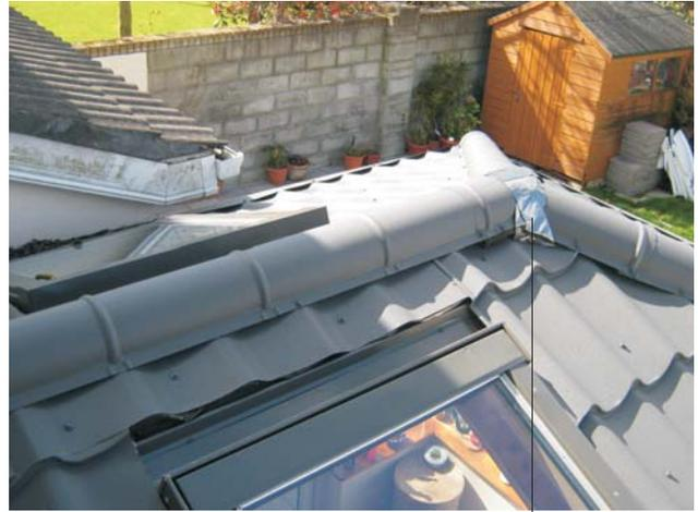
Adhesive tape flashing peeling from capping junction
