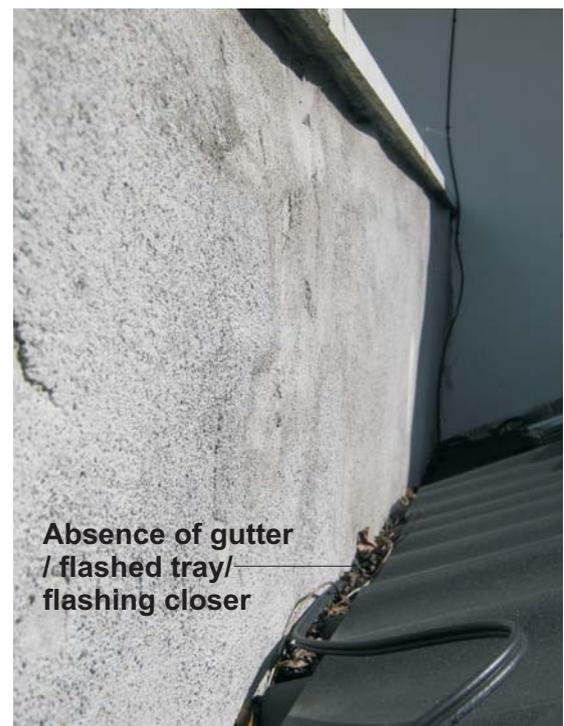
**Photo looking in at parapet wall**
