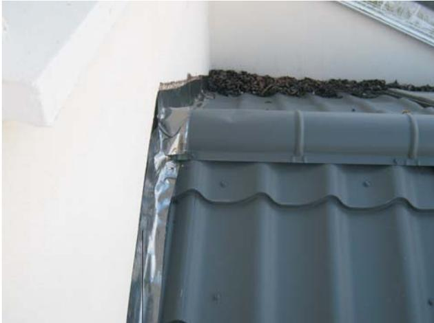
Adhesive tape flashing peeling off wall
